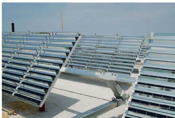
Figure 4: JX Crystals Inc 4 kW installation in Shanghai (top) with 2 Array Technologies trackers with 12 mirror panels per tracker. (Bottom left:) Photo of panels on 100 kW installation. (Bottom right) Panel power yields with average at 190 W and high of 205 W.
